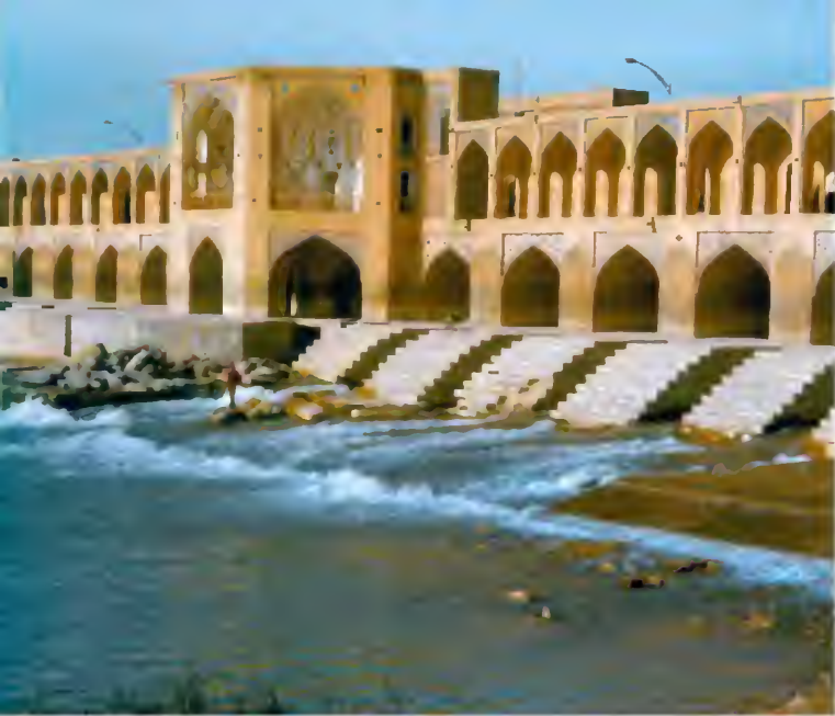
Khaju Bridge, also a dam, on the River Zayandeh in Isfahan, Iran was built in the mid 17 th century by Shah Abbas II of the Safavid dynasty. The bridge was set on a stone platform and divided by sluices which regulated the flow of the river.
